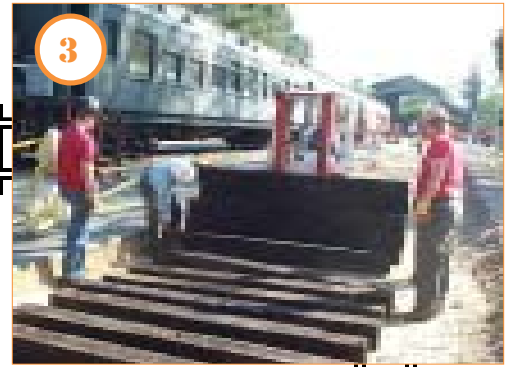
3 April 2: Volunteers lay out new cross-ties on the graded right-of-way.
