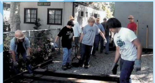
Laying out the ties for the 1940s track panel.
