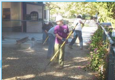
Preparing the site.
