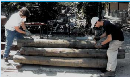
Using hatchet and drawknife, Owen and crew prepared "rough log ties" for the 1860s-era track panel.
