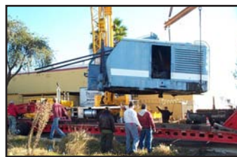
8:54 a.m.: Now separated from the car body, the machinery house is turned 90-degrees and loaded onto a waiting 9-axle truck.
